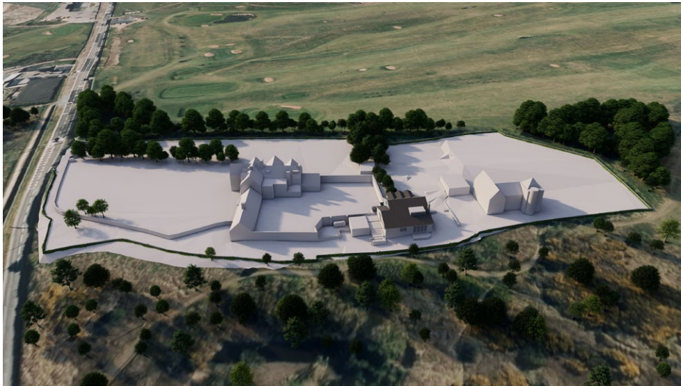
Existing view (looking south towards Whitburn Golf Course)
